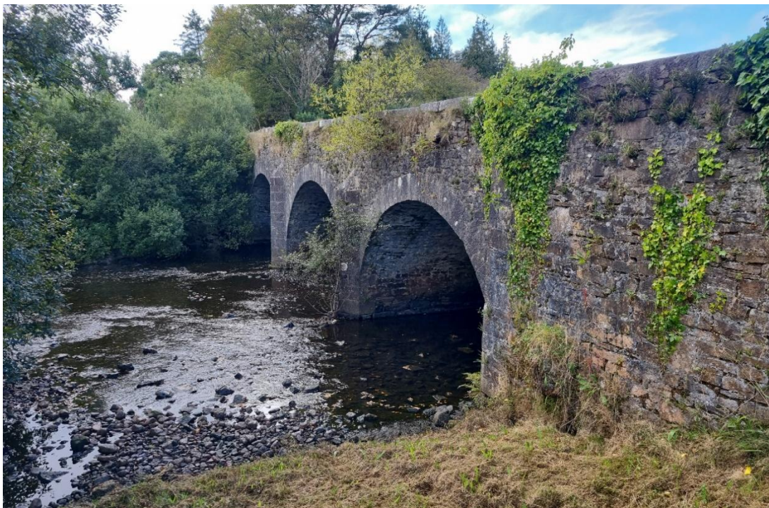
Figure 2-3 - Existing Road Bridge over River Eske (S05)
