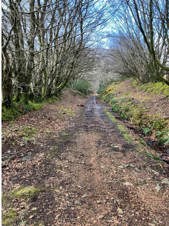
Figure 2-4 - Abandoned Railway Corridor
