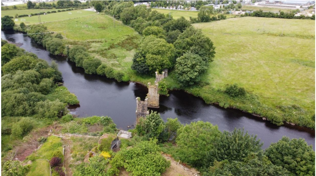
Figure 2-7 - Existing Railway Piers in River Finn
