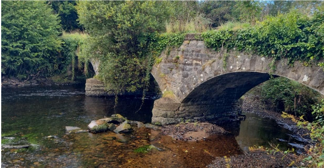
Figure 2-1 - Existing Railway Bridge Structure at River Eske in Donegal Town
